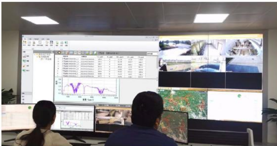
Central control screen
